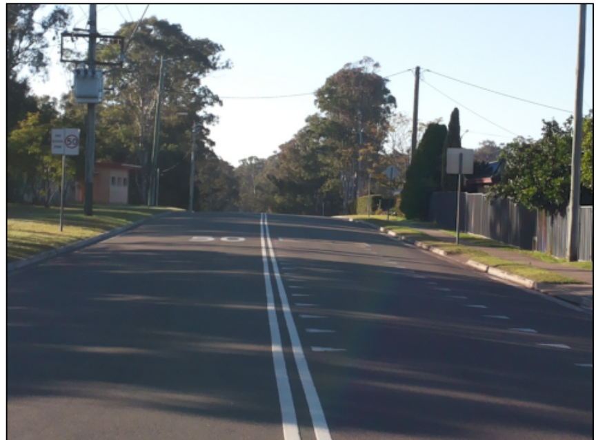
Figure 2.8: Littlefields Road – Looking east from Mulgoa Road
